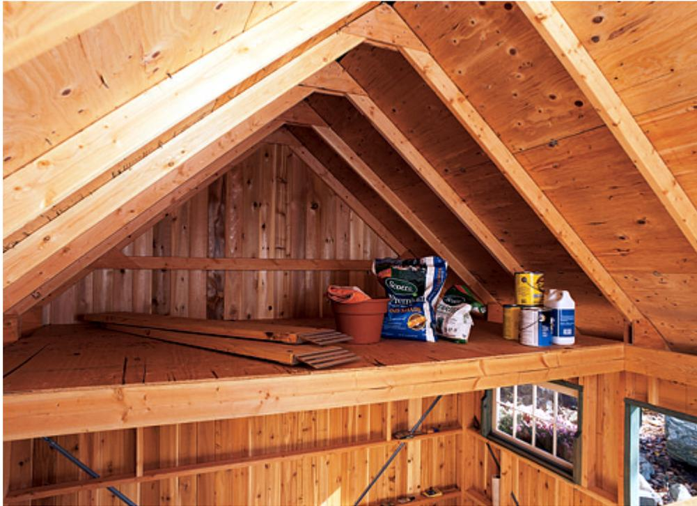
If you choose, you can customize the shed by creating a small storage loft at one or both ends. Here, the 2 x 6 chords of central trusses are cut away after assembly and their cut ends are framed across. Then, a plywood deck is installed
