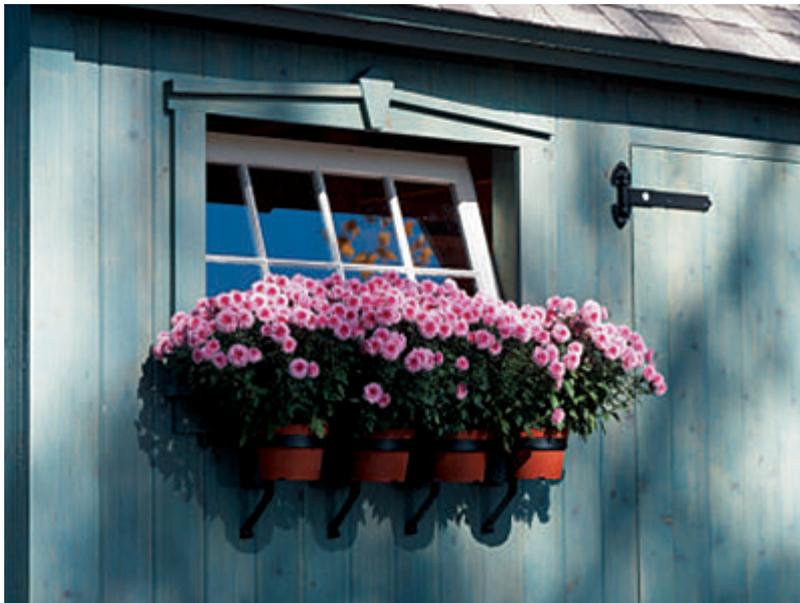
Barn-sash windows pivot at the sides to allow for ventilation. Siding, doors and trim are made of cedar.
